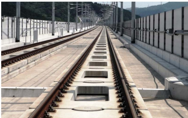
Figur 3.3 Frame slab track (Japan).
