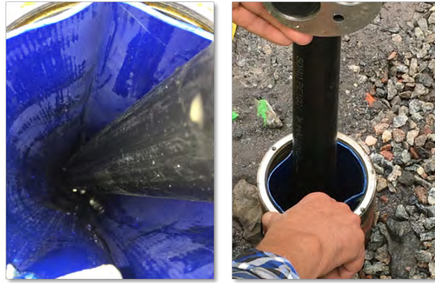
Figure 5.3: Pictures of the coaxial borehole heat exchanger during installation
