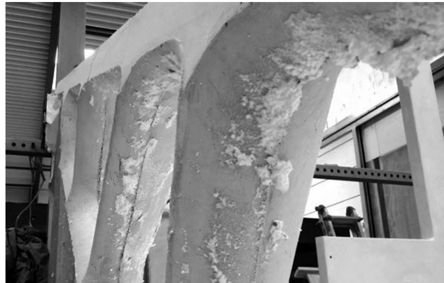
FIGURE 1.17 An illustration of the adhesion of high-performance concrete to an expanded polystyrene mould (Hi-Con, 2017) (Source: Hi-Con A/S).
