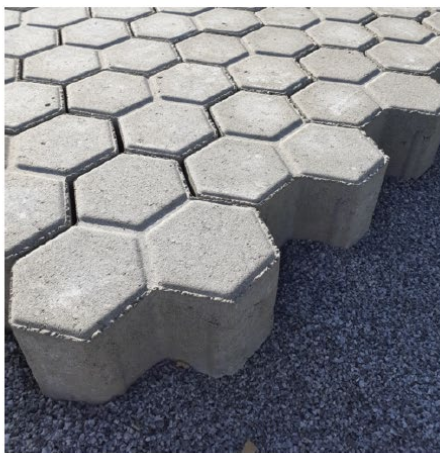
Figure 1a: Norvik Port concrete Trihex pavers on asphalt
