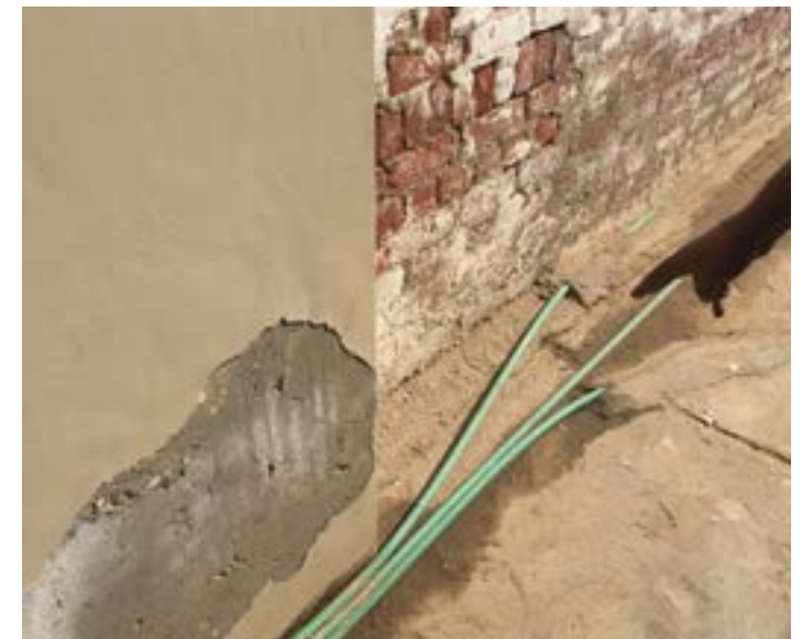
A section of an informal piped water supply network made in Rwata, a peri-urban village on the outskirts of Delhi, India. Photo: Timos Karpouzoglou.
