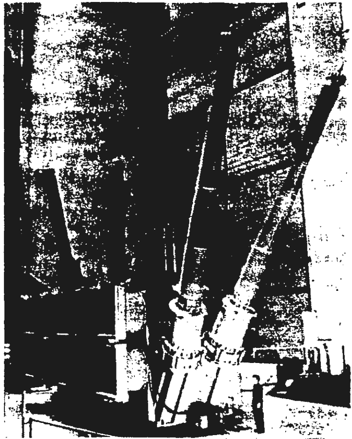
Figure 1-18 a) 12-pulse converter with three single-phase three-winding converter transformers and three quadruple valves. b) Single-phase three-winding transformer for the Intermountain Power Project (IPP).
