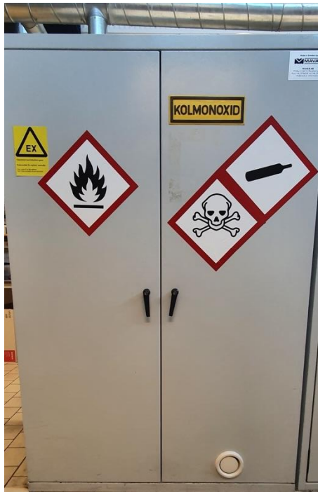
Figure 4: Example of an approved, fire-resistant gas cylinder cabinet required for flammable gases (EN 14470-2 standard).
