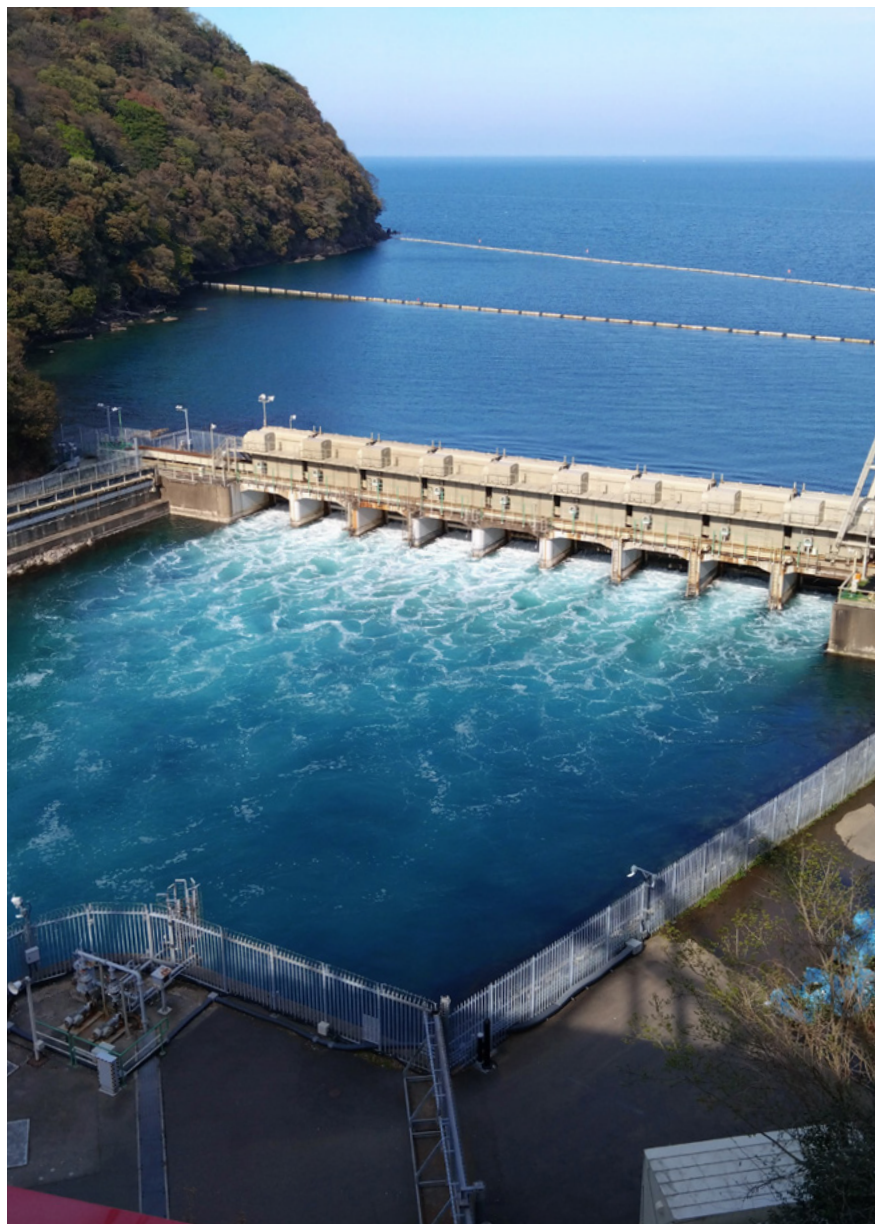
Cooling water inlet at the Takahama nuclear power plant. Seawater from the Sea of Japan is flowing by gravity into the lower-lying power plant area.
