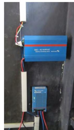
Figure 10 : Inverter and charge controller
