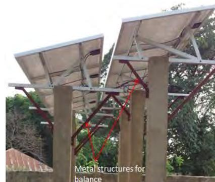
Figure 9 : Structure reinforcement
