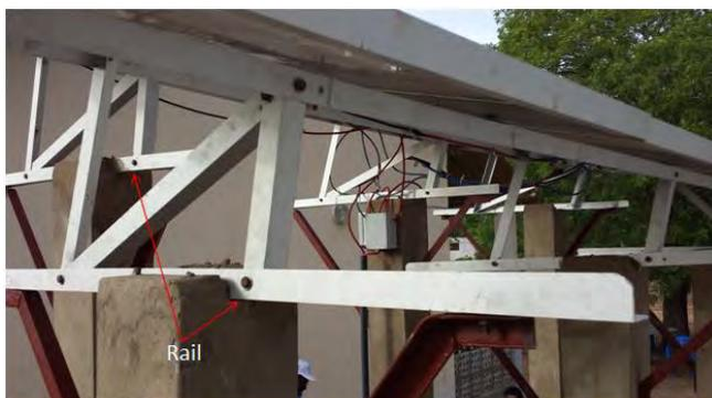
Figure 8 : Fixation to the pillars
