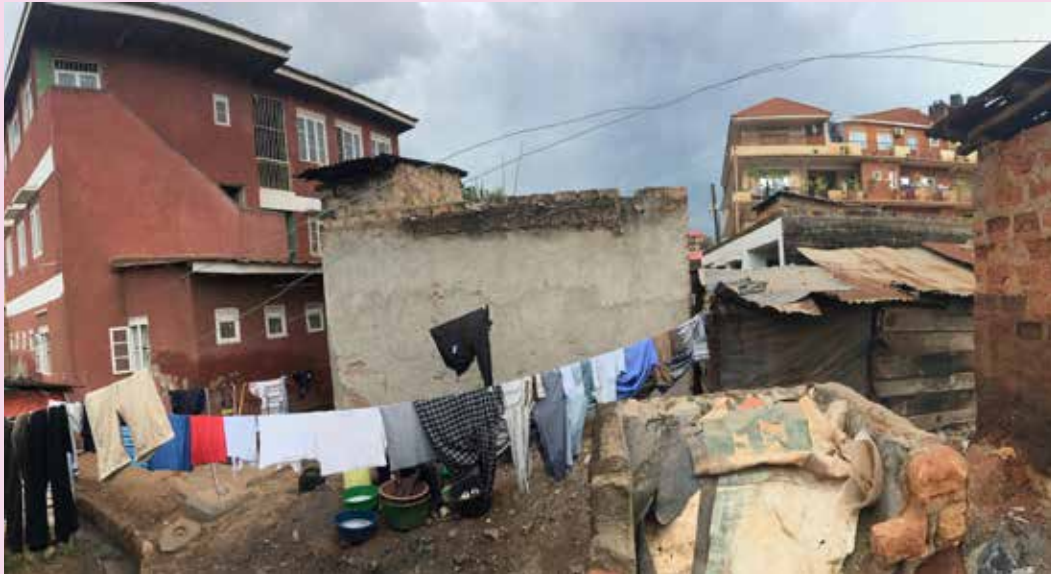
The urban heterogenous infrastructure landscape of Kampala, Uganda, shows two different types of toilets. To the right a dug pit latrine with a brick structure. To the left a pink three-story building that houses a community-toilet and bath which has been funded by the local neighborhood and built by a local branch of the Slum Dwellers Federation. The top two floors are used as a community space for meetings and during the days, as a school. Photo by Henrik Ernstson, 2017.
