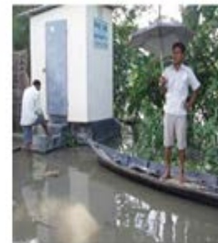
Raised toilet, Bangladesh
