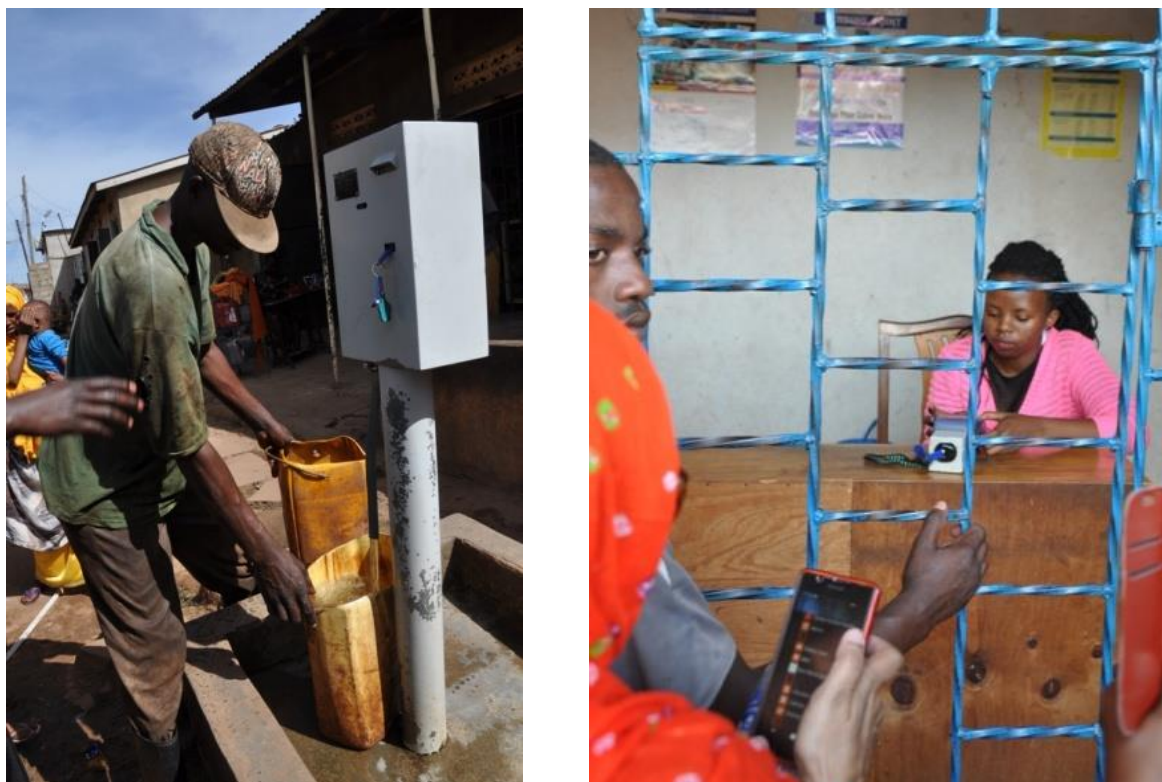
Figure 3 (a) pre-paid water dispenser in Kisenyi, Kampala; (b) sales point for water credit. Photo: David Nilsson
