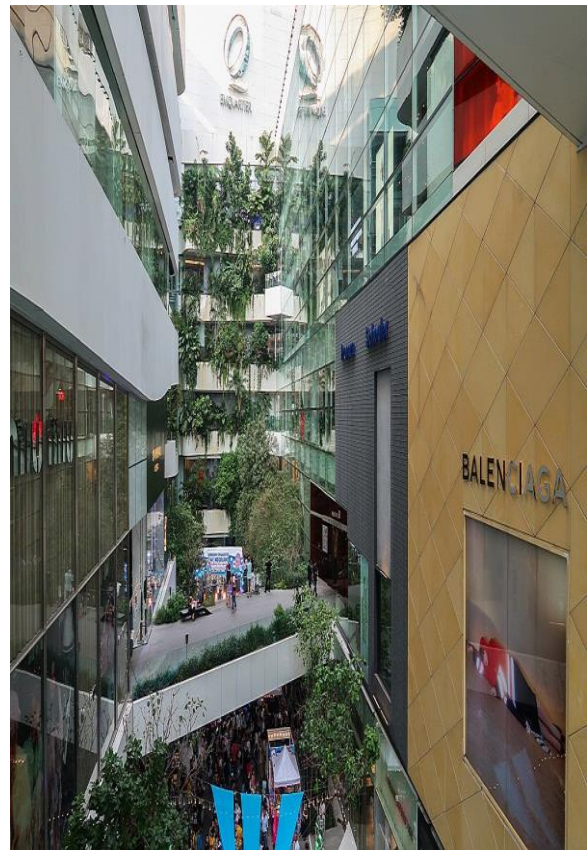
Figure 20. Floating gardens scattered across multiple stories.
